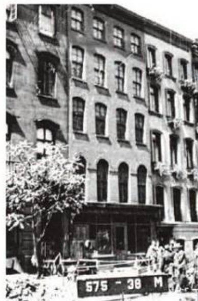
SF Vanni at 30 12th Street 1940
